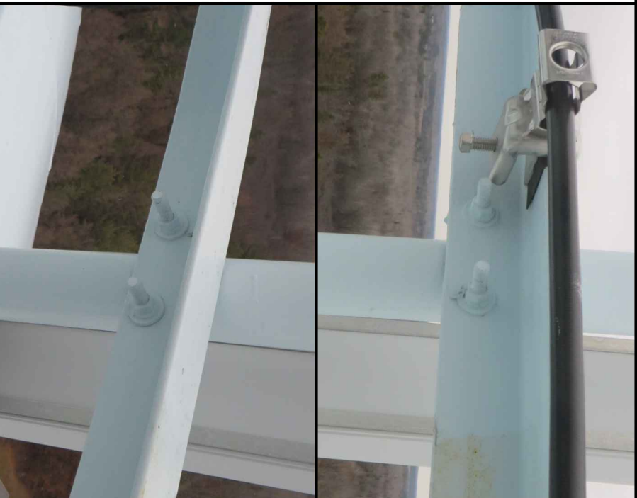
EXISTING MAST PIPE MOUNT
