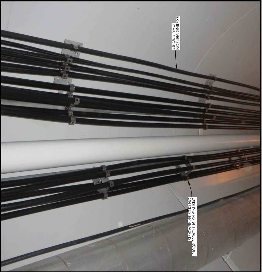
LOOKING UP TANK SHAFT
